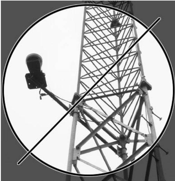
Receiver on Radio Tower
